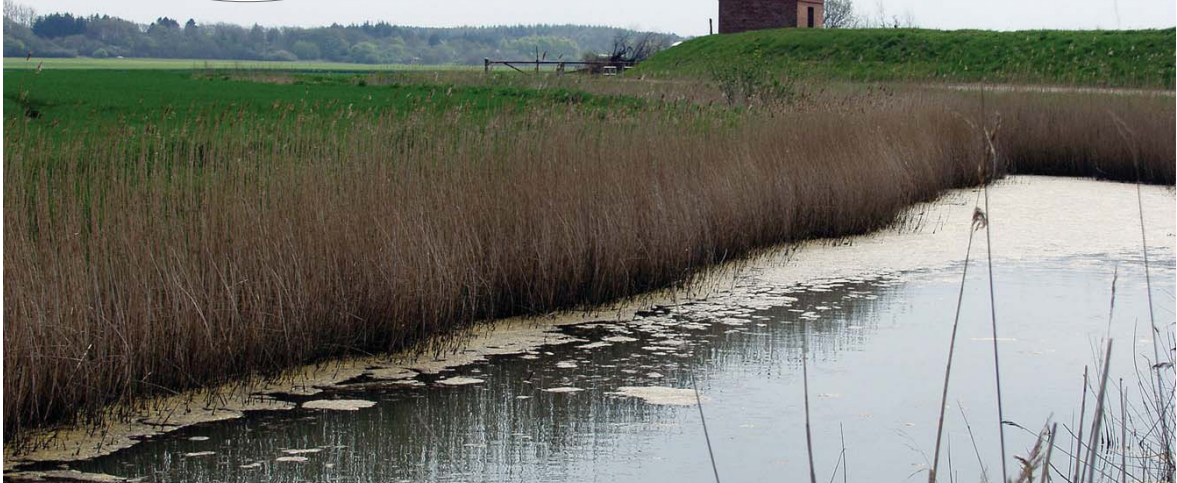
Pumpehus, Kahr Holme Digelag
